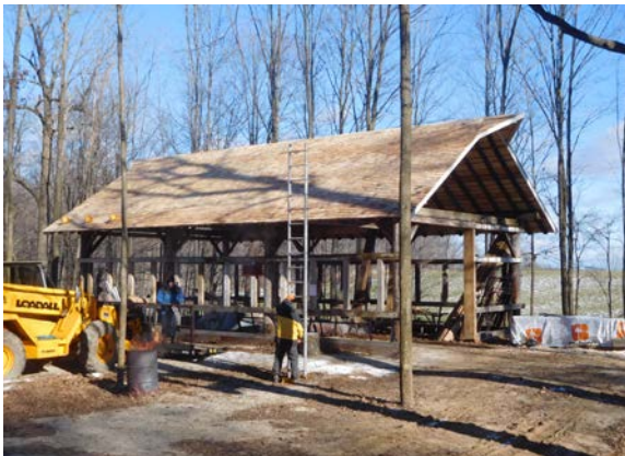
Blacksmith Shop under Construction
