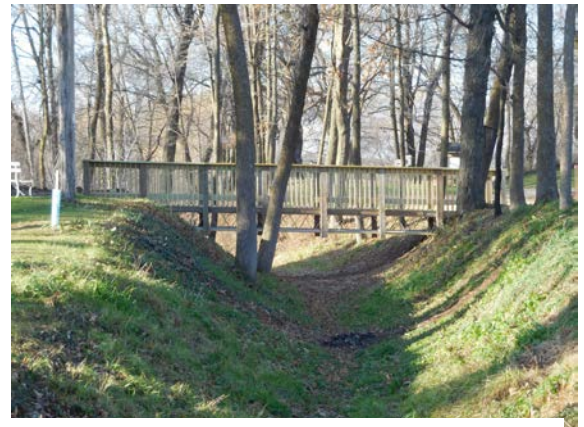
Bridge Connecting Mill House and Welcome Center
